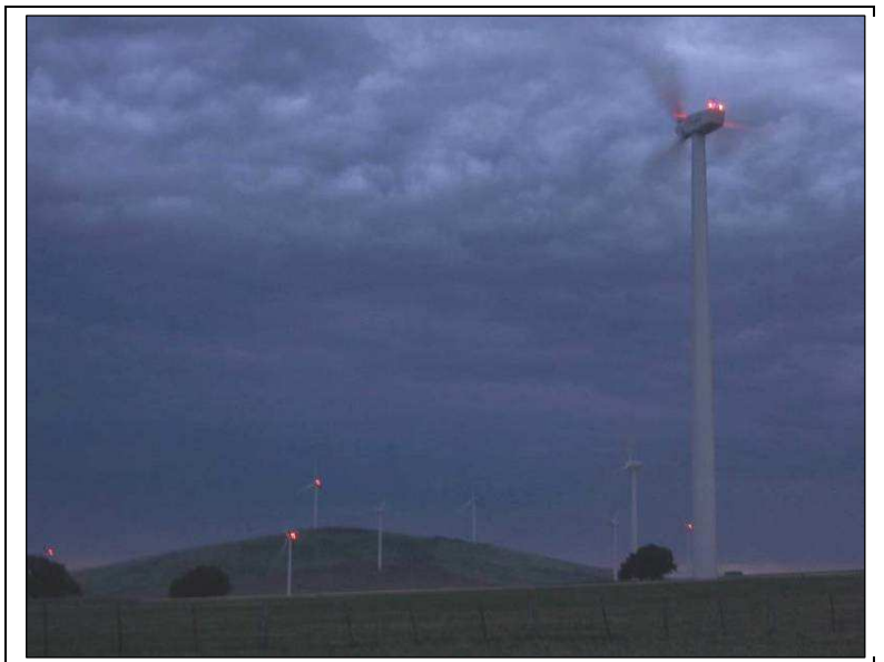
Photo 2: Warning lights and visual effects, blades emphasised by the lights
